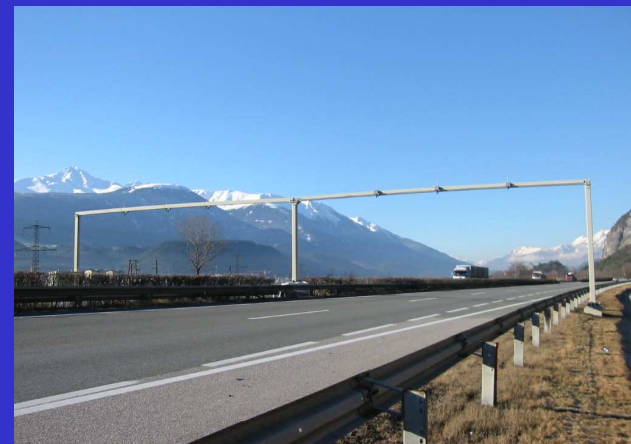
more than 800 Toll Gantries
